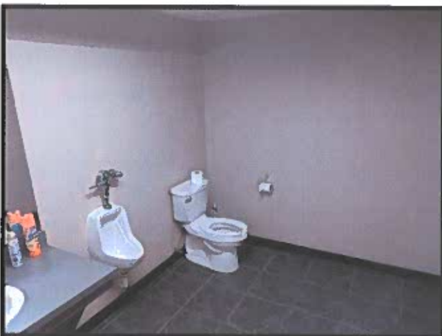
Parks/PW Dept. Restrooms, No Safety Handle
