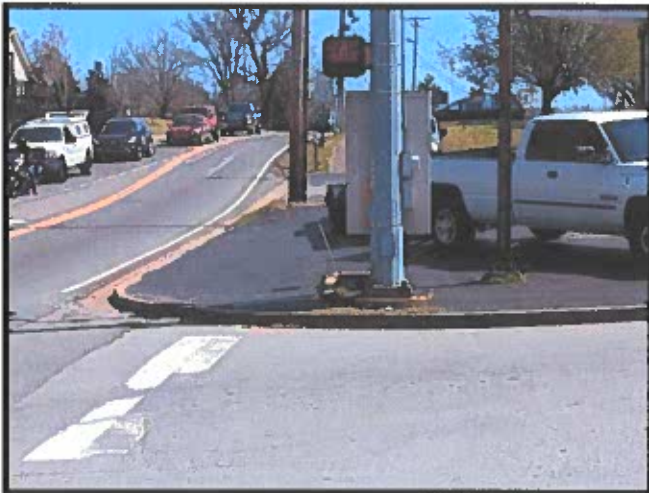
Main St. and Stratton/Elizabeth Signal Pole without ramp or Crosswalk
