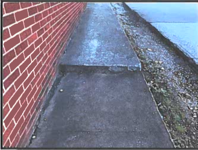
North Vine Street- Changes of Level, Step-ups
