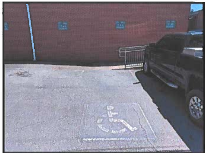
Example Faded or No Signage
