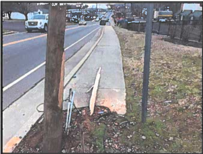
Main Street/HWY 12 Utility Pole Obstruction and No Clear Path
