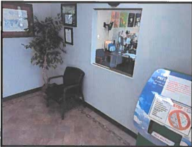
Police Dept. Window Counter Too High
