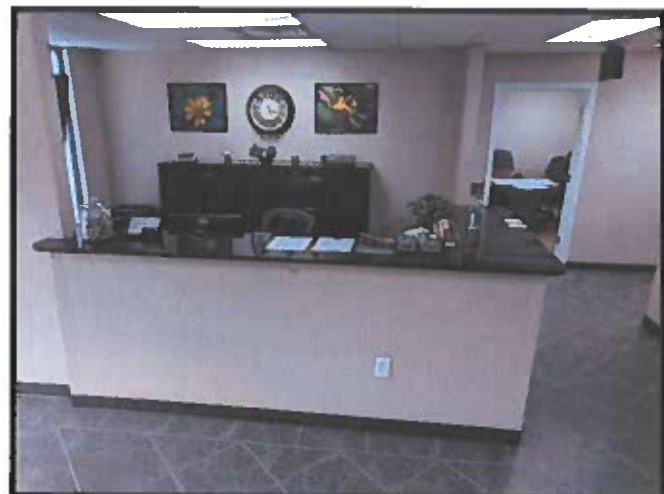
Parks/PW Dept. Service Counter Too High
