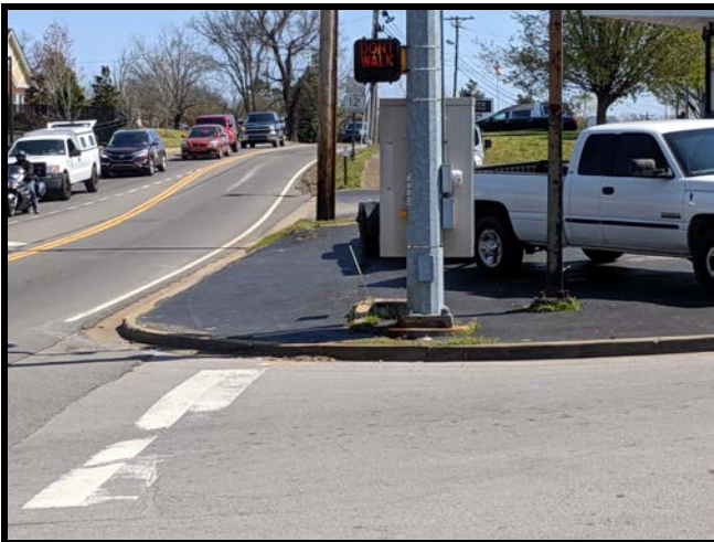
Main St. and Stratton/Elizabeth Signal Pole without ramp or Crosswalk
