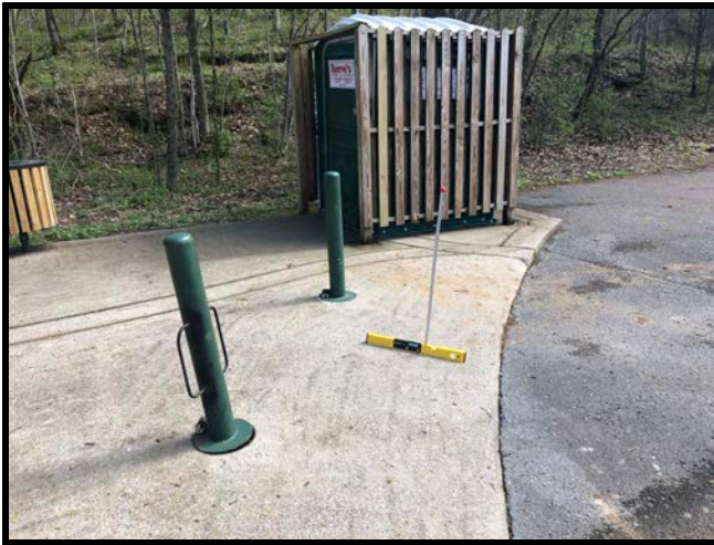
Bicentennial Trail Eagle Pass Trailhead-Ramp Slope
