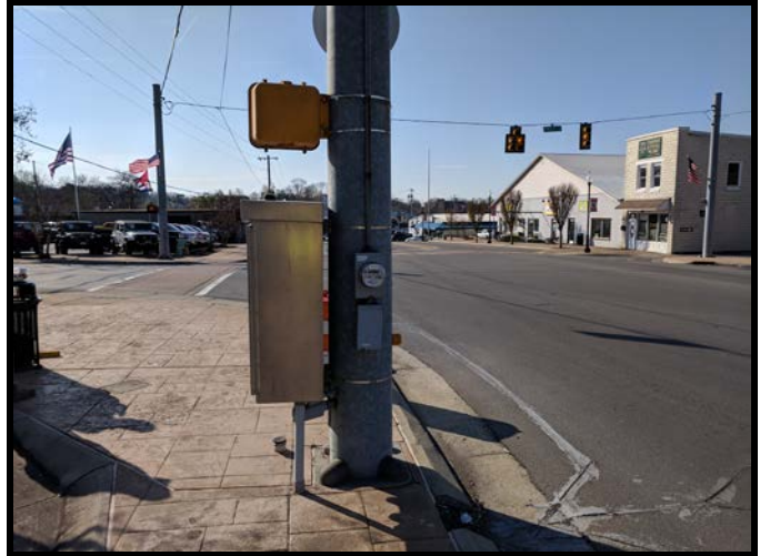
Main St. and HWY 49/Frey St. Pushbutton on Street Side and >30' from Crosswalk
