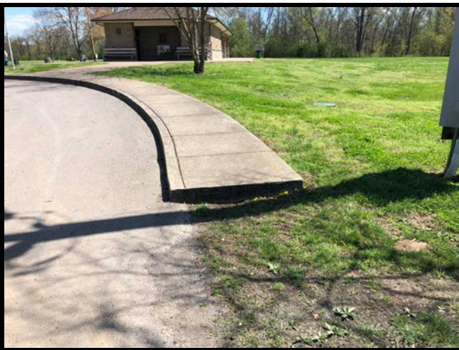
Riverbluff Park, Sidewalk End
