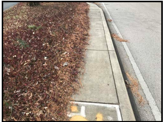
Helen Street- Typical Obstruction Due to Overgrowth
